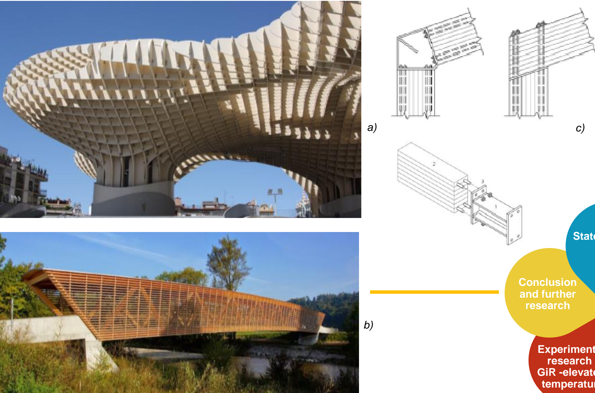
Figure 1: a) Glued-in rods as a connection method in long-span timber structure - Metropol Parasol in Seville, Spain; b) Neumatt Bridge, Switzerland - joints in the timber truss were made using GSA® technology developed by neue Holzbau AG; c) Application of GiR in moment-resistant joints
