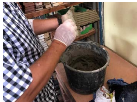
Figure 4: Adding mortar on the
