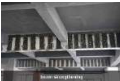
Figure 1: Beam strengthening
