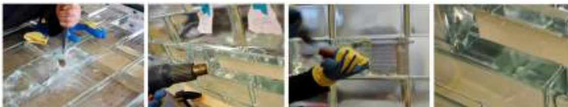
Figure 1: De-bonding method using heat developed for the Crystal Houses Façade
